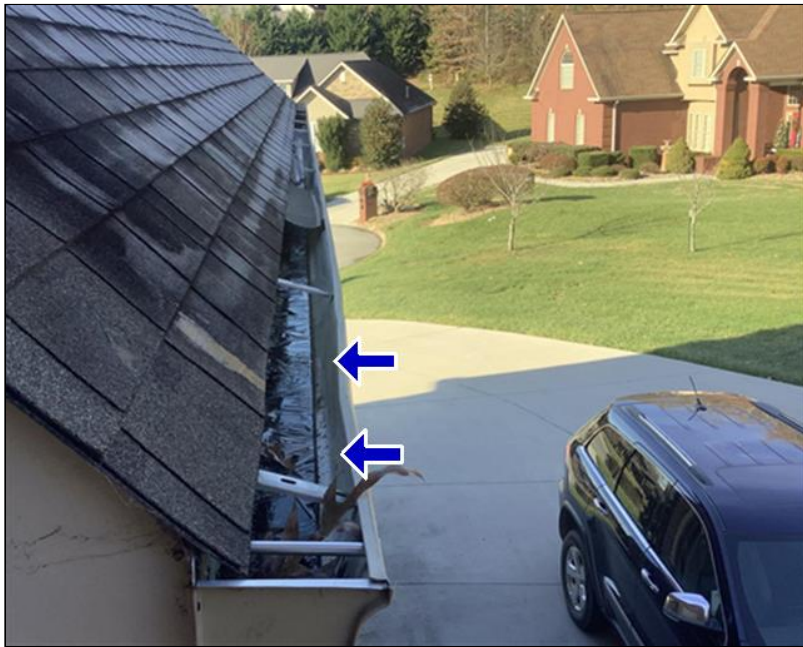
1.4 Item 1(Picture) Gutter over garage
