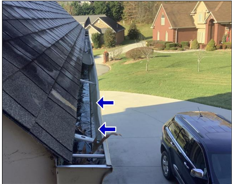
1.4 Item 1(Picture) Gutter over garage
